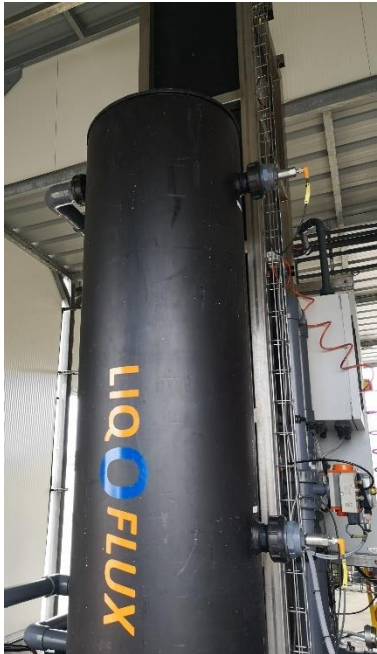
Filtration 0.5 - 2 m 3 /h
